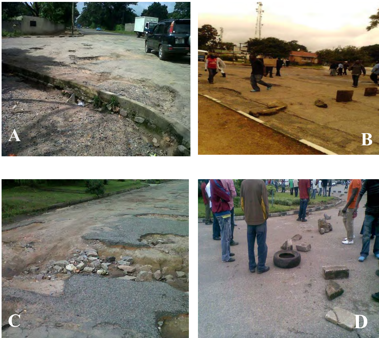
A and C show the poor state of roads in Chingola. B and D show residents blocking roads during a protest in Chingola. Source: Mubanga Chileshe and social media
